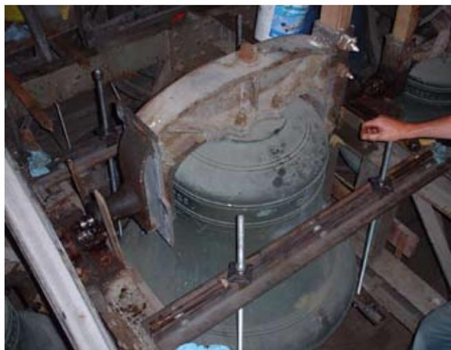
*The tenor bell lifted up awaiting the new bearing to be fitted. Bell to left is treble, right is the 4th.*
